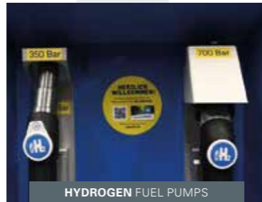
HYDROGEN FUEL PUMPS
